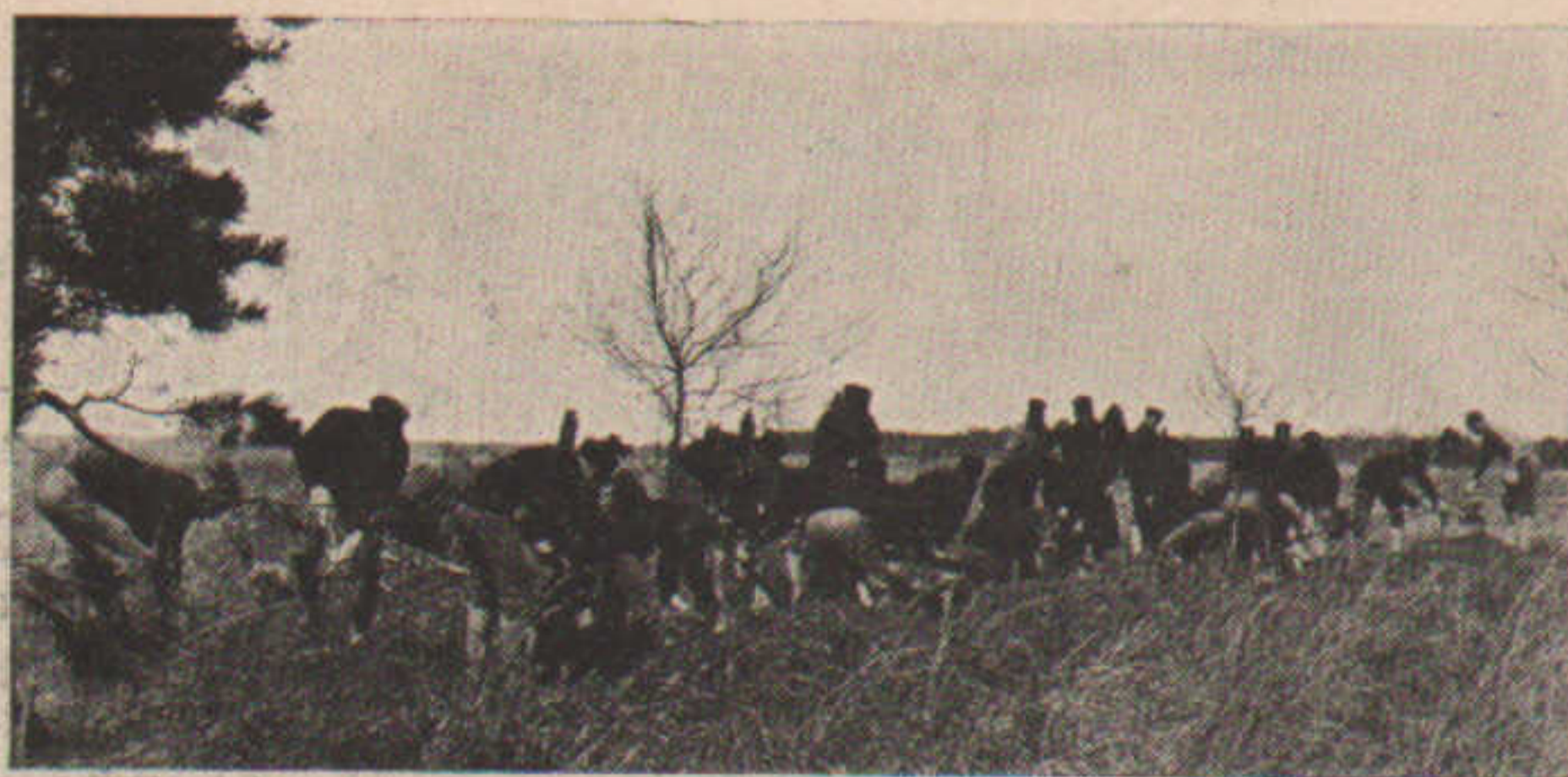
CUT N.—OFTEN INTRENCHING MUST BE DONE IN CLOSE QUARTERS.
