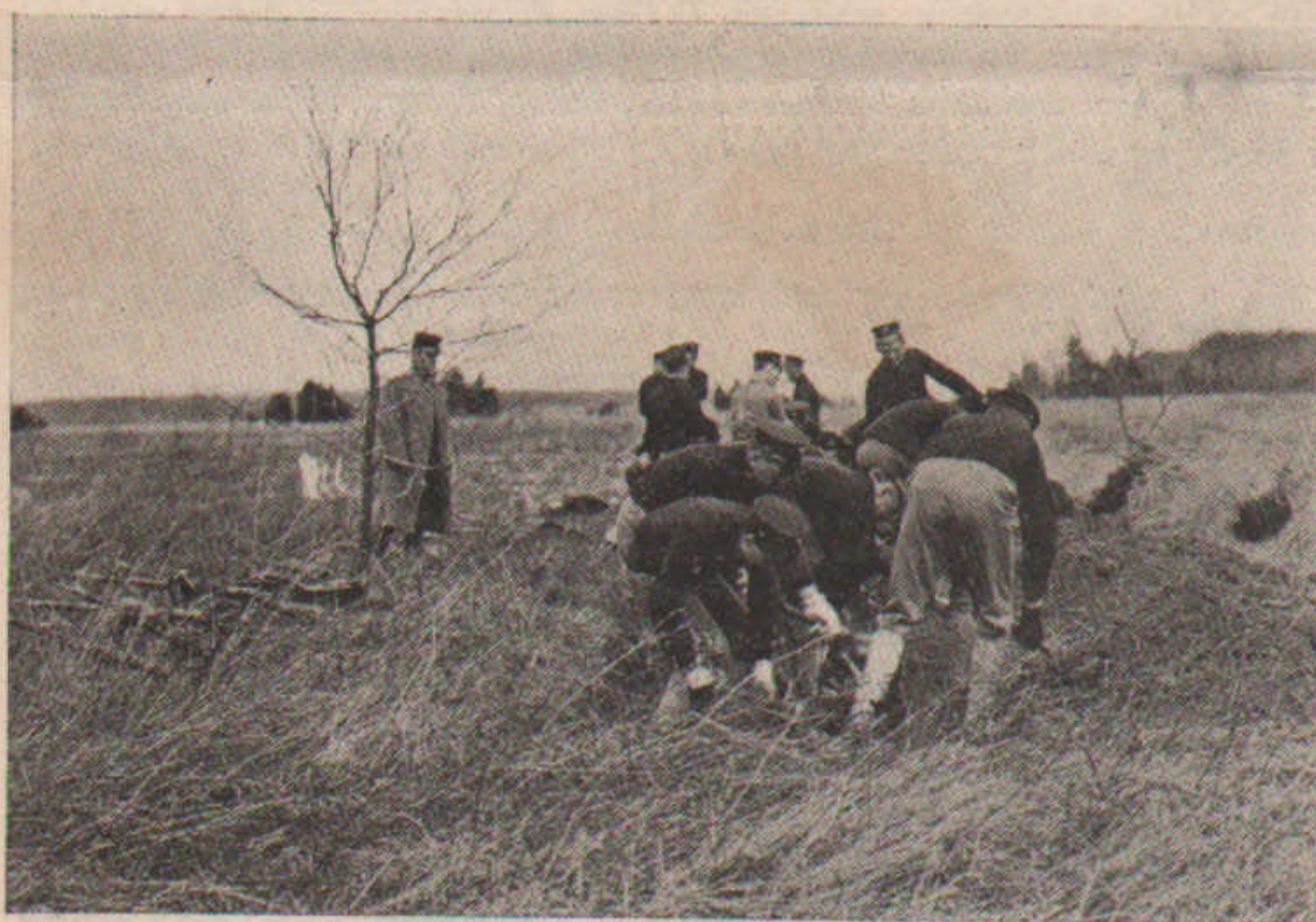
CUT O—A SHORT-HANDED INTRENCHING TOOL IS A CONVENIENCE.
