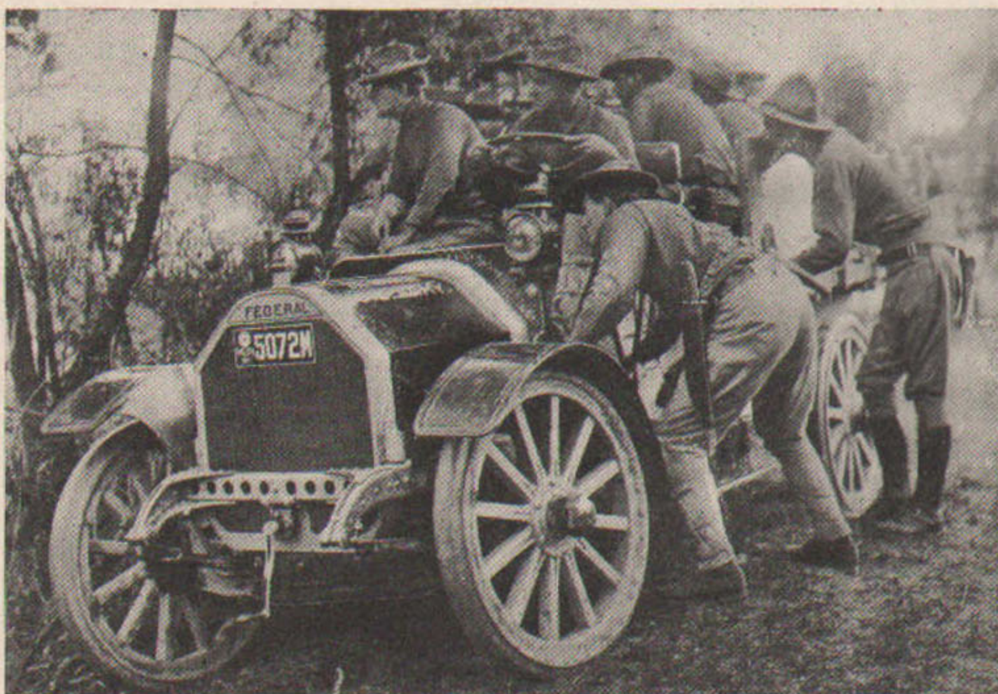
Machine Guns Screened—Ready to Open Fire.
