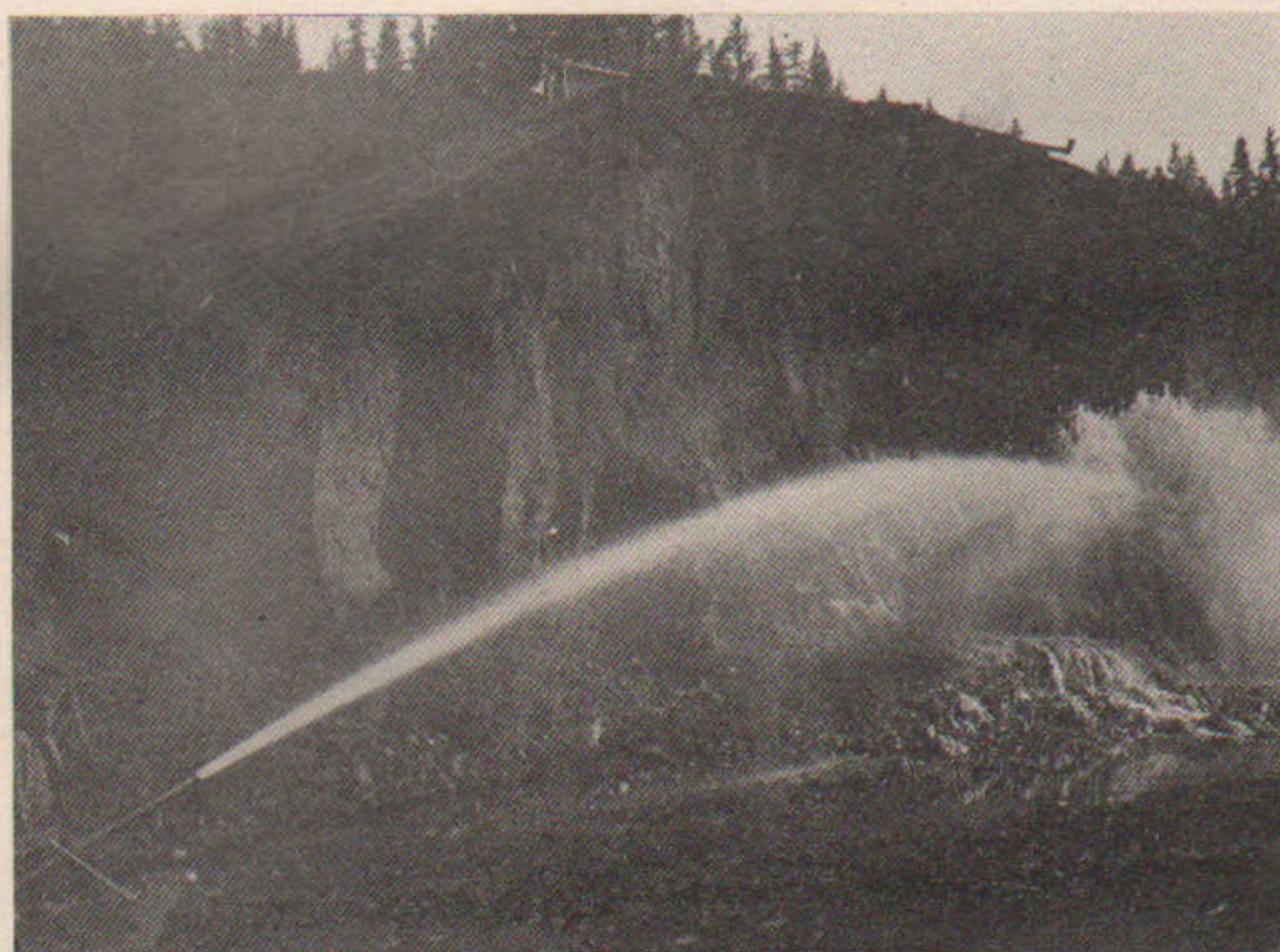
The Bank and the Stream That Did the Work.
