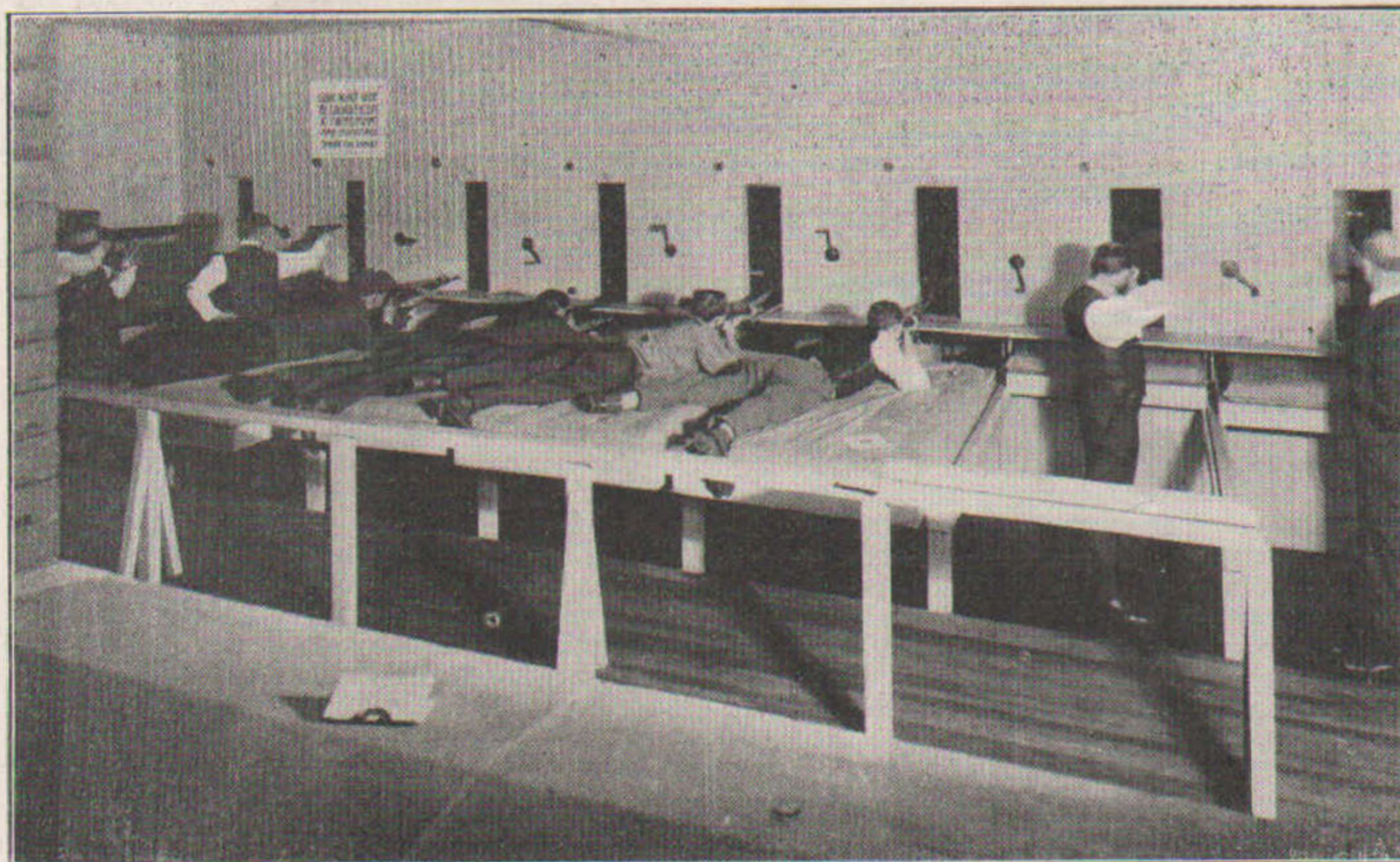
Firing Line of the Roof Garden Range Showing Individual Openings, Target Control Levers, Prone Platforms and Standing Pits
